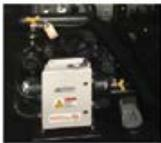
UL listed jacket water heater with isolation valves comes standard
